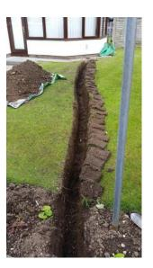
4. We will provide the ducting - lay this in the trench making sure that it's reasonably straight and is not going to be damaged by sharp stones. Consider sieving the soil back over the duct or laying it in some sand.
